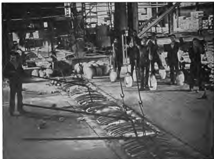
FIG. 111.—One of the melting furnaces used for making crucible steel. (Courtesy of the Crucible Steel Company of America.)
